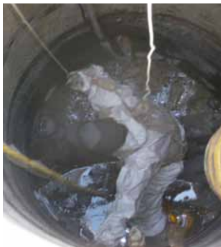
Left: Pump ragging & clogging is a problem everywhere and can lead to constant rebuilds and disruption of pump stations. Right: Operator installs the waste grinder in a tight fit to clear out debris.
