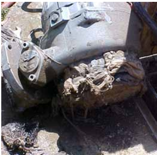
Left: Pump ragging & clogging is a problem everywhere and can lead to constant rebuilds and disruption of pump stations. Right: Operator installs the waste grinder in a tight fit to clear out debris.
