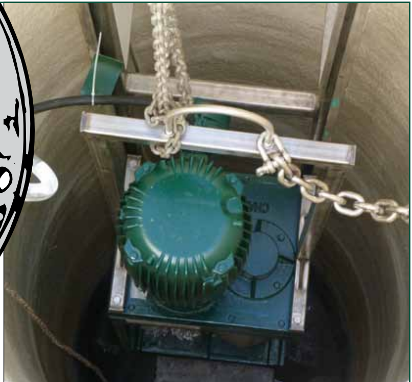
The Channel Monster, custom fitted for Santa Ana manhole, slides down a guide rail for an easy access sewage grinder. (credit: Brian Ige, P.E., City of Santa Ana)
