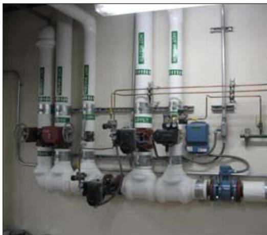
**The new biogas-heated hot water loop has ancillary branches to heat the building, front walkway, and headworks washwater.**
