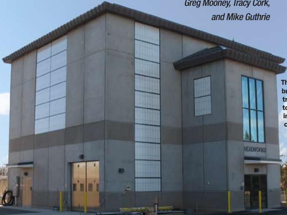
The new headworks building uses translucent panels to let natural light in while reducing cleaning requirements.
