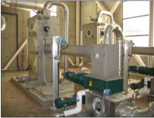
**The liquid stream is completely enclosed to contain odors and harmful gases.**
