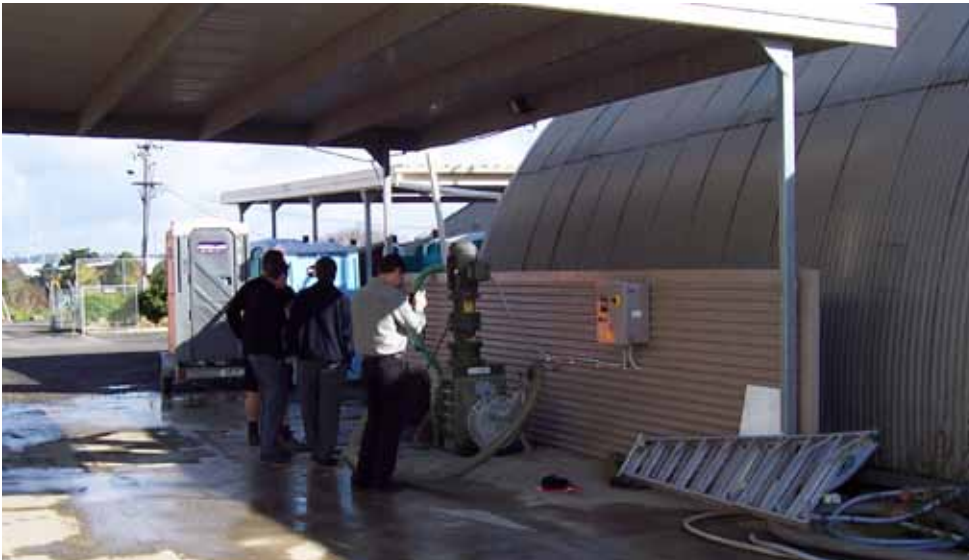
Operators inspect the Monster which grinds solids and septage unloaded from their trucks.
