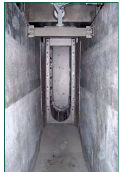
The Bandscreen Monster, installed in November 2005 as part of the JWC Monster Separation System.
