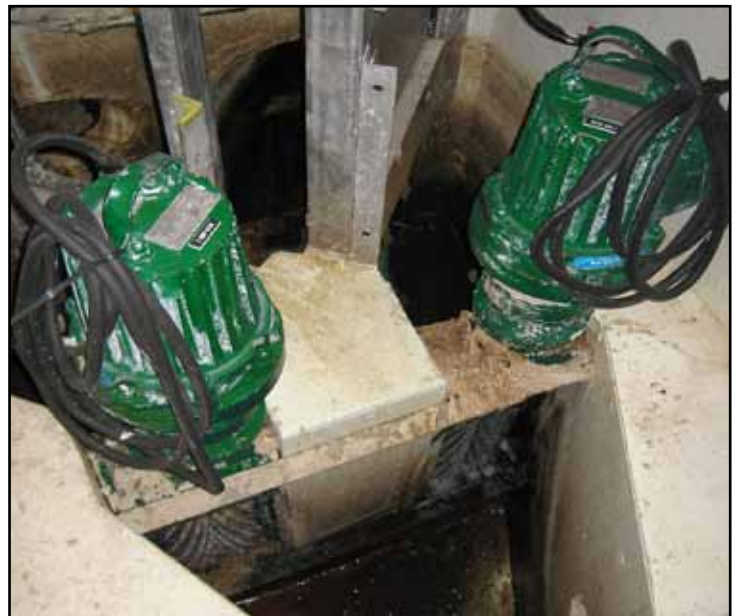
Equipped with immersible motors, these Monsters are protected from high flow levels so they can devour the debris in the wastewater.
